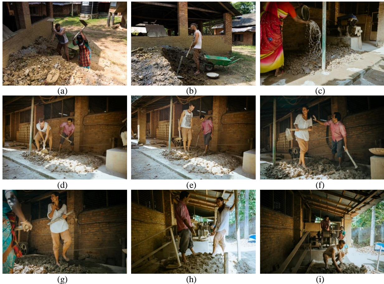
Fig. 2 Traditional clay preparation [19]
